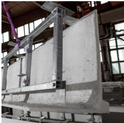
installing fixing system
